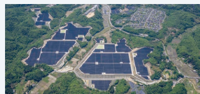
Large-scale solar power generation facility that straddles Kyoto-Mie prefectural border
