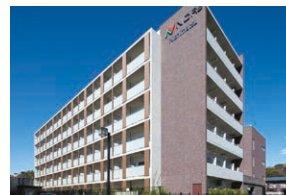
Managed by Nishimatsu Construction, Keio University Hiyoshi International Dormitory was recertified by JHEP
