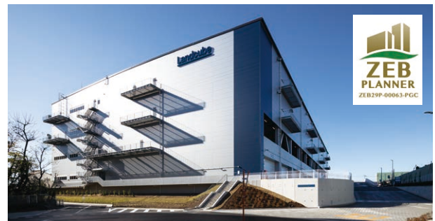
Landcube Ageo (warehouse, steel construction, four above ground stories, total floor area: 39,859m 2 )
