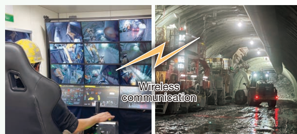
On-site tests for the wheel loader remote-control system (Tunnel RemOS-WL)
