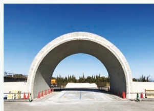
Completed development pouring for renewed lining technology
