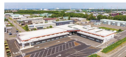
Panorama of the Ishikari Shinko Nishi Construction Project. Award Theme: Proactive 3R activities for construction work in a large-scale industrial park subject to various restrictions
