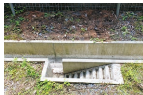
Gutter staircase for small animals (Kanto Civil Engineering Regional Headquarters, Minami Koma Worksite Office)
