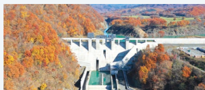
Dam body construction at the Biratori Dam
