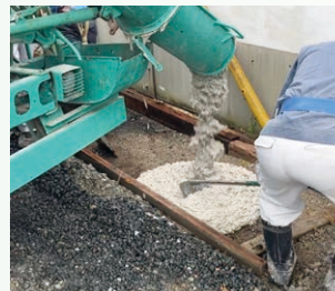
Placing (agitator car's shoot)
