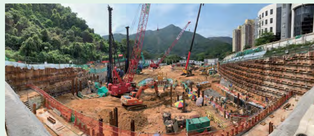
Overall view of Fu Shan Public Mortuary site
