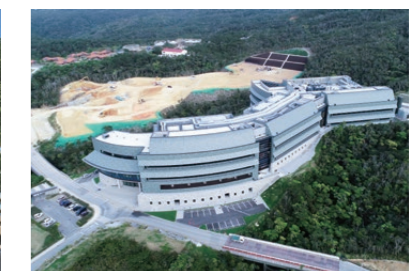
Okinawa Institute of Science and Technology Graduate University Building 4 and Other Construction Project Client: Okinawa Institute of Science and Technology Graduate University
