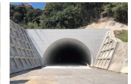
Okunohira Togitsusen Prefectural Road Improvement Works (tentative name: Kururi Tunnel)
