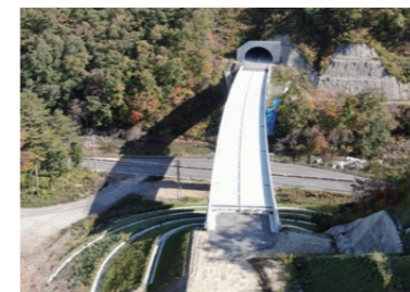
National Route 45 Hagyu-kita District Road Works
