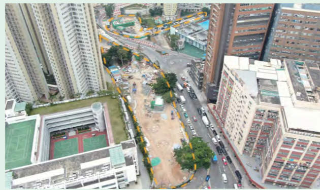
Aerial View of DOS site adjoining San Po Kong Public Housing Development
