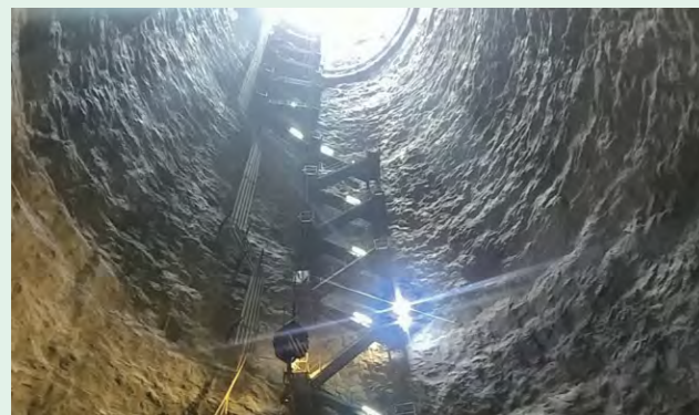
View from the bottom of completed Ho Man Tin Access Shaft
