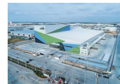
Construction of Frasers Unicorn factory Client: Frasers Property (Thailand)
