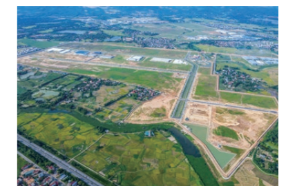
Thang Long Industrial Park III Phase 2 and 3 grading and infrastructure works Client: Thang Long Industrial Park (Vinh Phuc)
