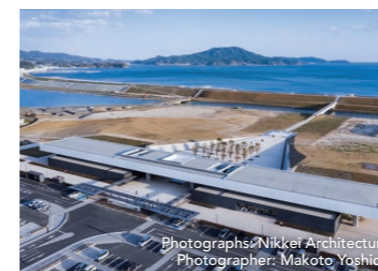
Takada Matsubara National Memorial Facility (tentative name) Management Building Construction Project Client: Tohoku Regional Bureau, Ministry of Land, Infrastructure, Transport and Tourism
