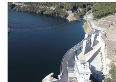
Fiscal 2016-2019 Yokozegawa Dam Body Works
