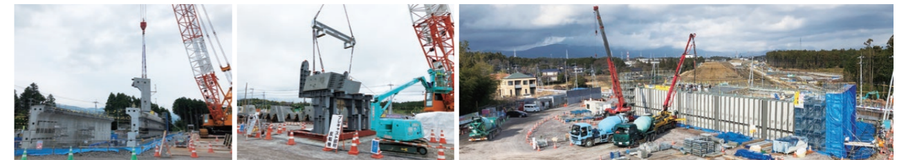
Installation of half-precast box parts
