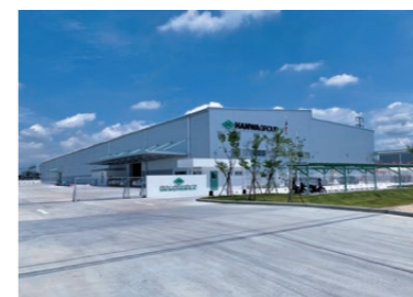
Construction of new factory of Hanwa Metals (Thailand) Client: Hanwa Metals (parent company: HANWA Co., Ltd.)
