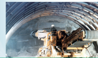
Seikan Tunnel (Sengen Construction Area)
