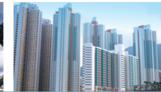
Aldrich Bay Residential Building, Phase 4, Hong Kong
