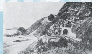
Hisatsu Line Construction Area No. 2
