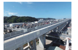
No. 3 South Fukui Viaduct
