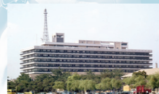
Otemachi Joint Government Building
