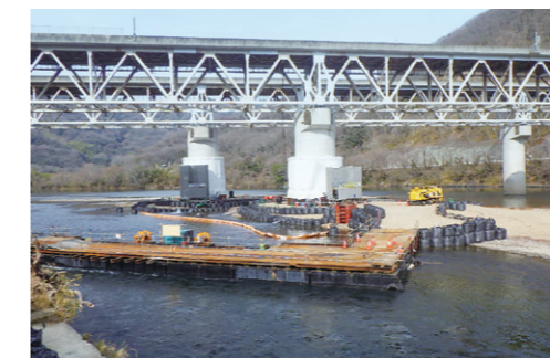
Floating type pier (front)
