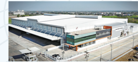
All New Complex Phase 2 Project
