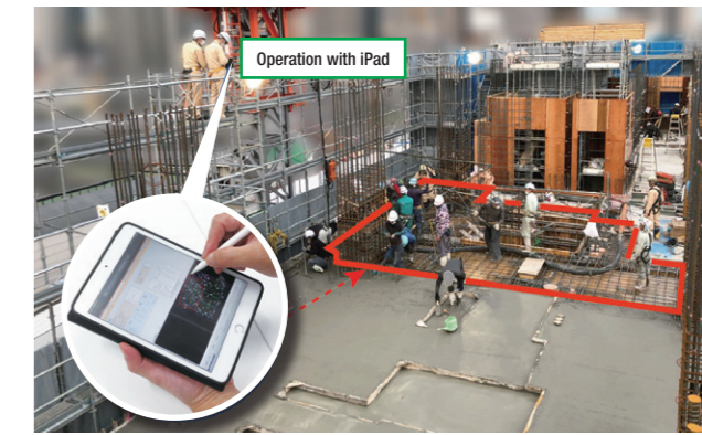
Automatic calculations can be performed by drawing a line around the required area on diagrams that are displayed on the iPad
