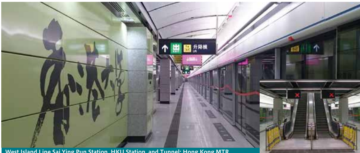
West Island Line Sai Ying Pun Station, HKU Station, and Tunnel; Hong Kong MTR
