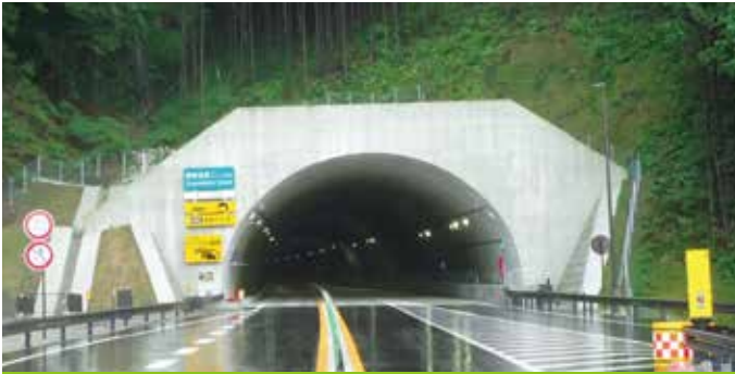
Susami No. 2 Tunnel Work, Kinki Expressway Kisei Route
