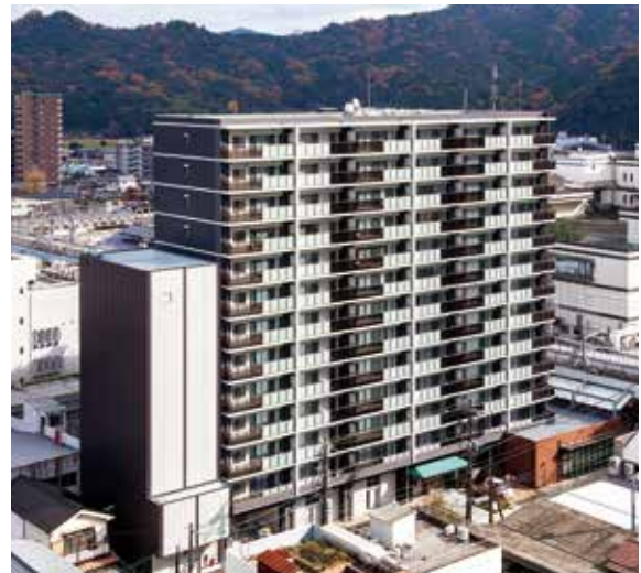
Yamaguchi Nakaichi-cho 1 (Building Complex Development Project)
