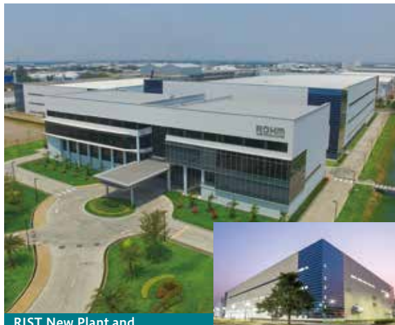
RIST New Plant and Welfare Building
