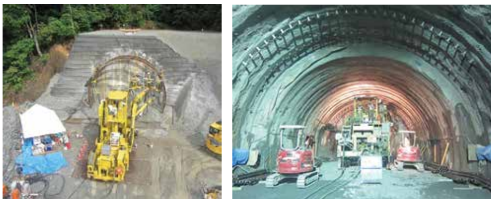
Real-life Working Scenes (L: Shaft entrance, R: Inside shaft)
