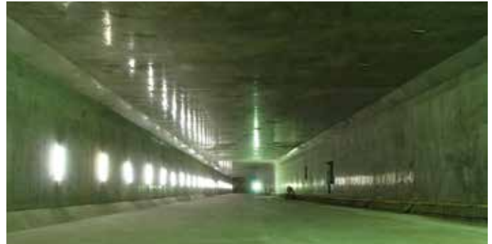
Kan-ni Underground Tunnel Construction (Shin-ohashi Area)
