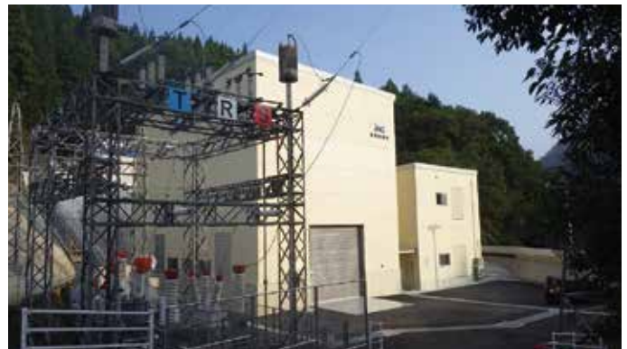
Kurino Power Plant Renovation
