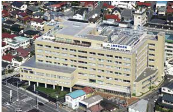
Kamitsuga General Hospital
