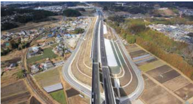
Shin-tomei Expressway Shinshiro Roadwork
