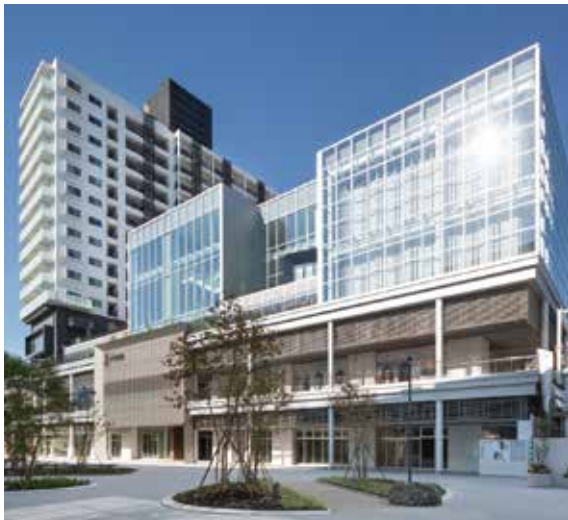
Tokai Otagawa Station West District (Urban Redevelopment Project)
