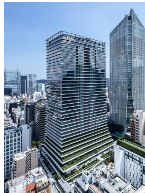
Toranomom Hills Business Tower
