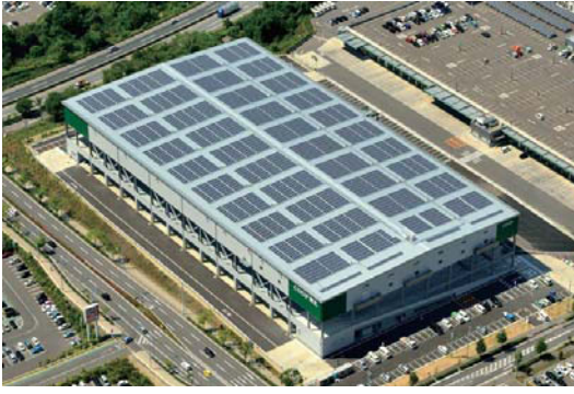
Coop Tohoku Dry Logistics Center Completed: June 2015 Location: Tomiya-machi, Kurokawa-gun, Miyagi Prefecture Total floor area: 42,970.60 m 2
