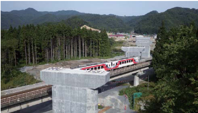
National Route 45 Omoto Roadwork
