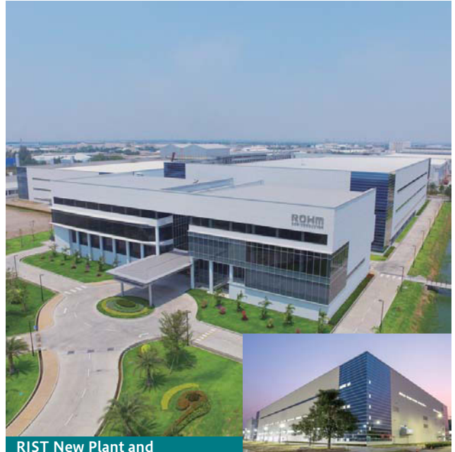
RIST New Plant and Welfare Building
