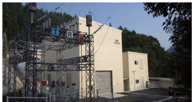
Kurino Power Plant Renovation
