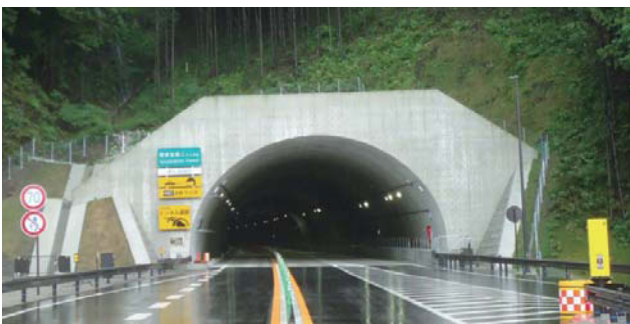
Susami No. 2 Tunnel Work, Kinki Expressway Kisei Route
