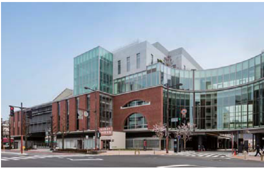
Kurume City Plaza Completed: November 2015 Location: Kurume-shi, Fukuoka Prefecture Total floor area: 10,829.90 m 2
