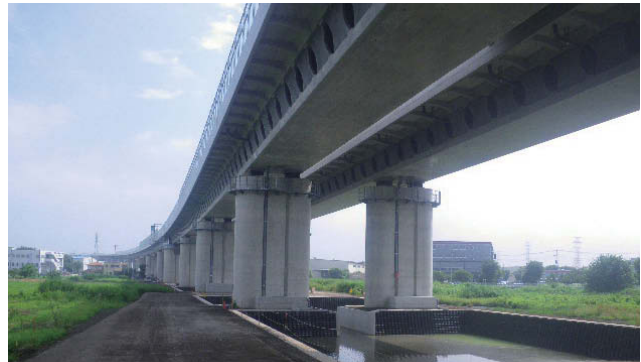
Okegawa No. 2 Elevated Bridge Substructure Work, Ken-O Expressway
