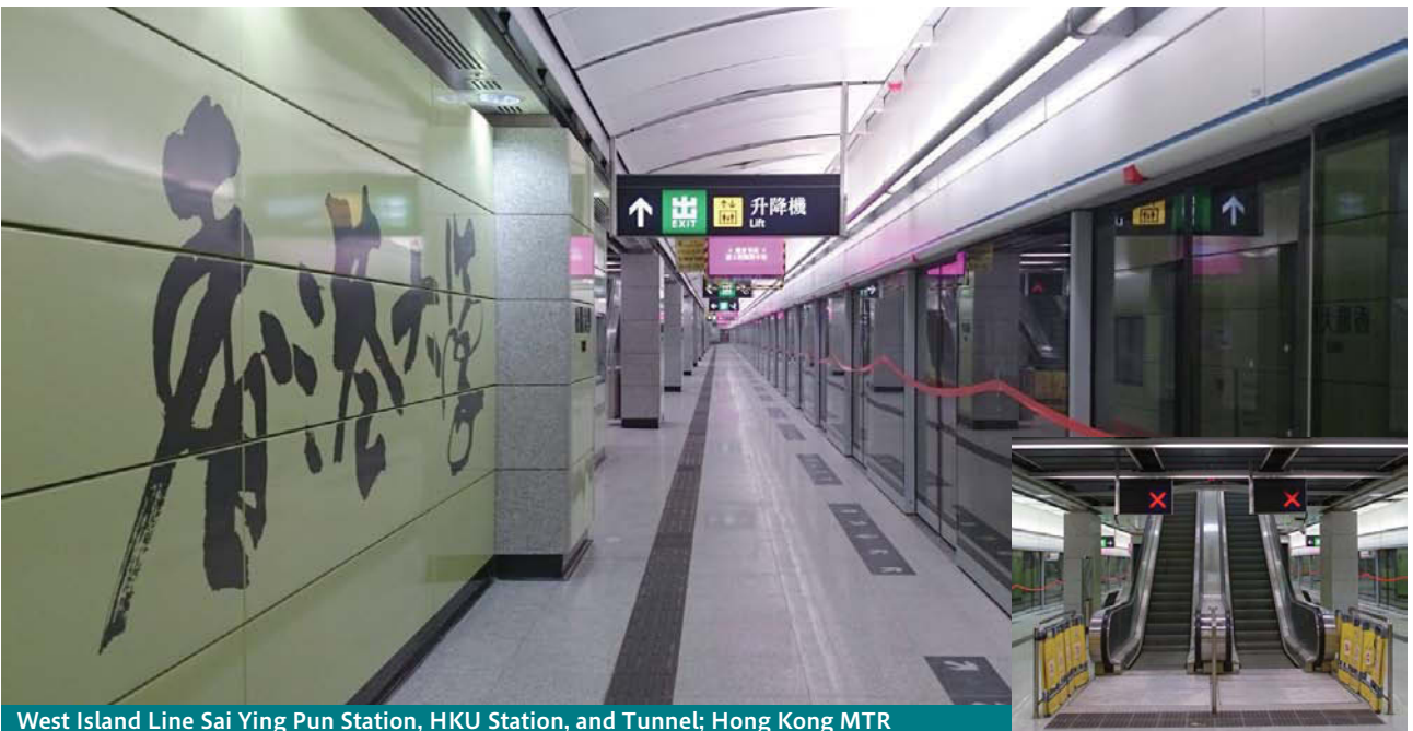
West Island Line Sai Ying Pun Station, HKU Station, and Tunnel; Hong Kong MTR
