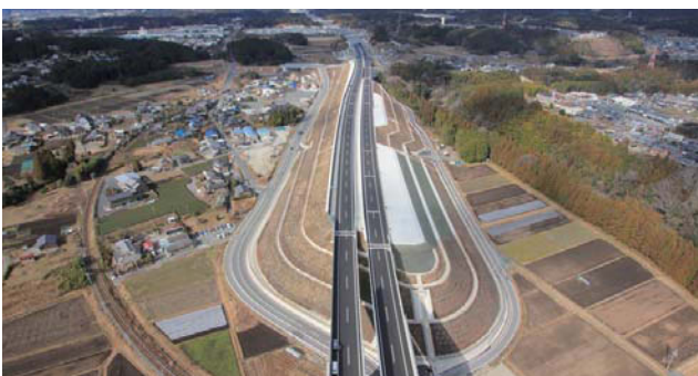
Shin-tomei Expressway Shinshiro Roadwork
