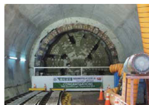
TBMs 1 and 2 reaching the May vertical shaft
