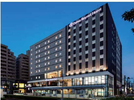
Daiwa Roynet Hotel Tokushima-ekimae Completed: September 2015 Location: Tokushima-shi, Tokushima Prefecture Total floor area: 9,170.54 m 2
