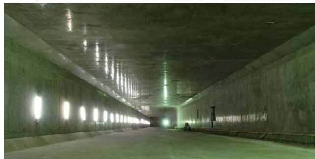
Kan-ni Underground Tunnel Construction (Shin-ohashi Area)
