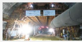
Automated set up of tunnel lining forms
