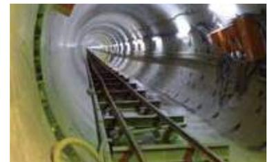
LED lighting inside shield tunnel construction sites
