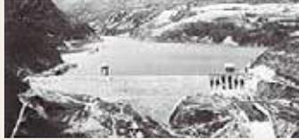
In the turmoil immediately following the end of World War II, this project was for a multi-purpose dam on the Isawa River in Iwate Prefecture. Since no precedent existed in Japan for this structure, Nishimatsu Construction relied upon reference documents from the U.S. and had to devise various creative solutions during construction.
