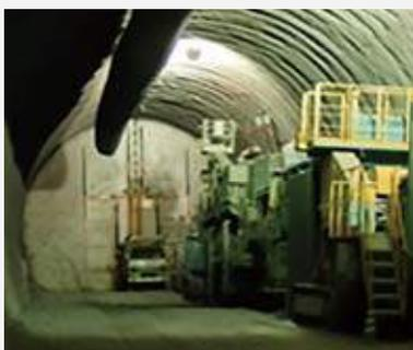
Portable blast protection balloon in use
