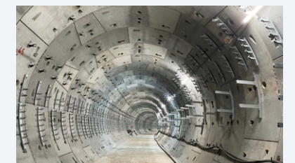
The Keppel Station tunnel on Singapore's subway Circle Line
