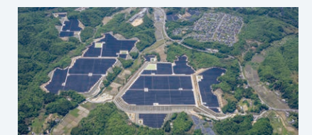
Large-scale solar power generation facility that straddles Kyoto-Mie prefectural border
