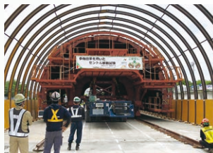
Slide form transport test using a multi-axis trolley
