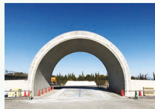
Completed development pouring for renewed lining technology
