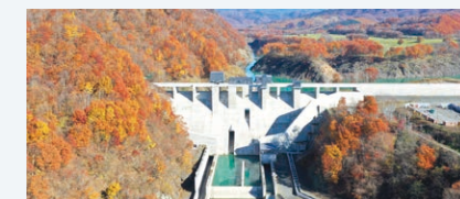
Dam body construction at the Biratori Dam
