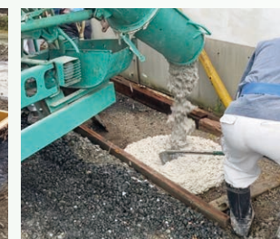
Placing (agitator car's shoot)
