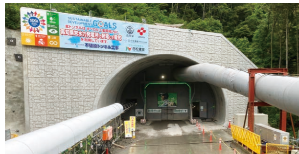
Tunnel construction site using renewable energy for 100% of construction power (Shikoku Branch, Fubahara Tunnel Branch Office)
