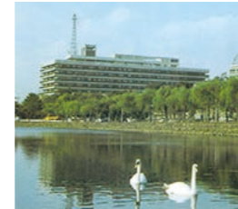
Otemachi Government Office Complex Building No. 1
