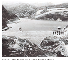
Ishibuchi Dam in Iwate Prefecture
