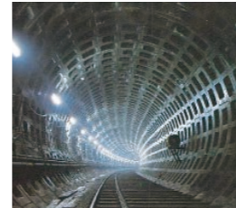
Keiyo Railway Line's Haneda-Oki Tunnel
