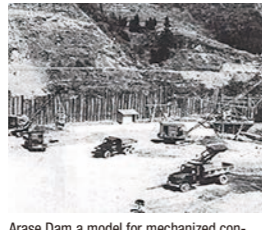
Arase Dam a model for mechanized construction site
