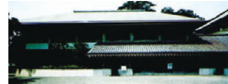
Japanese-style annex to the State Guest House
