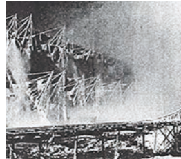
Galcheon Dam Under Construction During Winter (November 1935)
