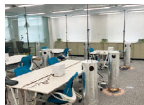
Air-conditioning performance test with simulated load
