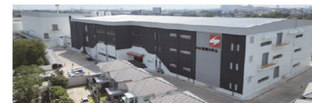
U.S. SANMINA's electronics and communications equipment factory expansion project (Thailand)
