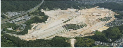
Hera Hill Development and Land Readjustment Project
