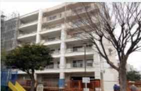
BiD frame construction
