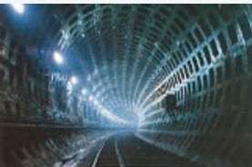
Keiyo Railway Line's Haneda-Oki Tunnel
