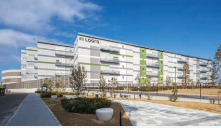
LOGI'Q Minami-Ibaraki [Project for Kurakakiuchi 1-chome, Ibaraki City, Osaka Prefecture] (tentative name)
