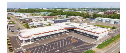
Panorama of the Ishikari Shinko Nishi Construction Project. Award Theme: Proactive 3R activities for construction work in a large-scale industrial park subject to various restrictions
