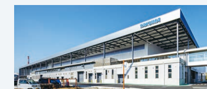
View of exterior on northeast side of factory
