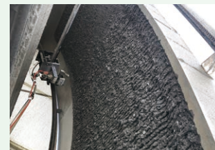
Water jet cutting was used to develop the technology to cut the existing lining
