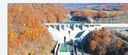
Dam body construction at the Biratori Dam
