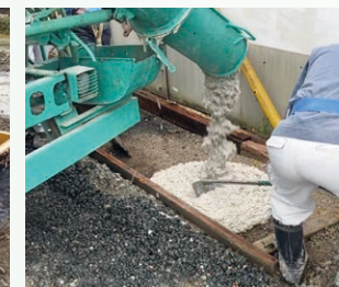
Placing (agitator car's shoot)
