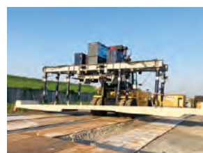
Full-scale transport and installation experiment using a large forklift and dedicated installation equipment
