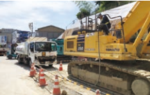
GTL fuel used in construction equipment (Kanto Civil Engineering Regional Headquarters, Kakio Site Office)
