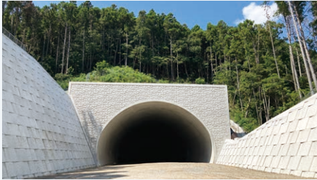
Construction work for establishment of the Matsuura 1st Tunnel route 497 in Nagasaki Prefecture
