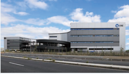
New construction of LogiSquare Fujimino A & B
