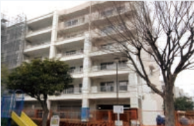
BiD frame construction
