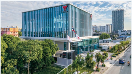
Yuasa Trading (Thailand) Co.,Ltd.'s new head office project
