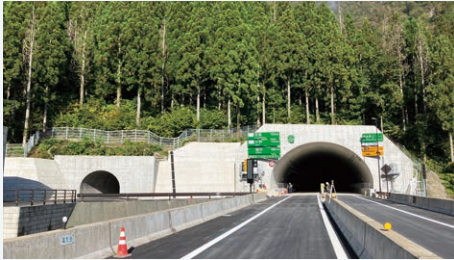
Construction work of the Arasima second tunnel area of Simoyama in Ono Aburasaka road
