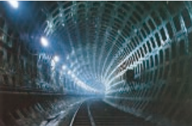
Keiyo Railway Line's Haneda-Okai Tunnel
