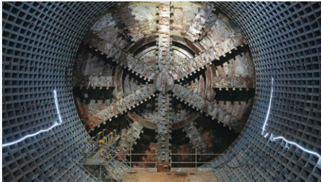
Yokohama Shonan Road Tunnel construction Phase 3
