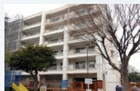
BiD frame construction
