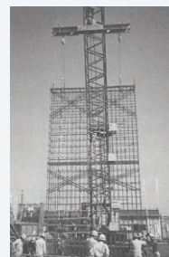
Deep continuous underground walls
