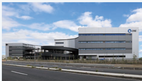
New construction of LogiSquare Fujimino A & B
