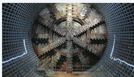
Yokohama Shonan Road Tunnel construction Phase 3
