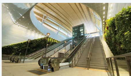
T228 Construction of Gardens by the Bay Station and tunnels for Thomson Line
