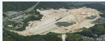
Hera Hill Development and Land Readjustment Project
