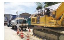
GTL fuel used in construction equipment (Kanto Civil Engineering Regional Headquarters, Kakio Site Office)
