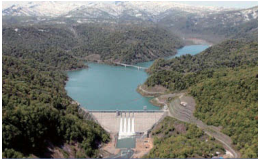
Kabato (Second Phase) Farm Irrigation Work Toppu Dam
