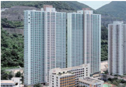
Construction of Public Housing Development at EX-Chai Wan Estate
