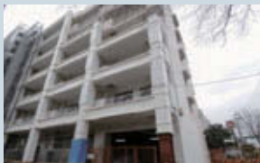
Full-size testing of BID (built-in damper) construction method
