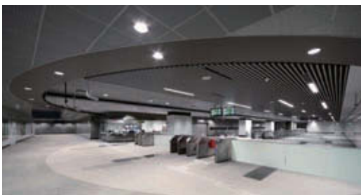
Contract C828, Design, construction and completion of stations at Nicill Highway & Stadium Stations including tunnels
