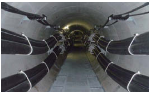
Suruga Higashi Shimizu, Abekawa Crossing Tunnel
