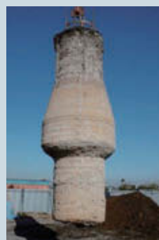
Diameter-expansion cast-in-place concrete pile. (Multi enlarged-nodes Ace pile method)
