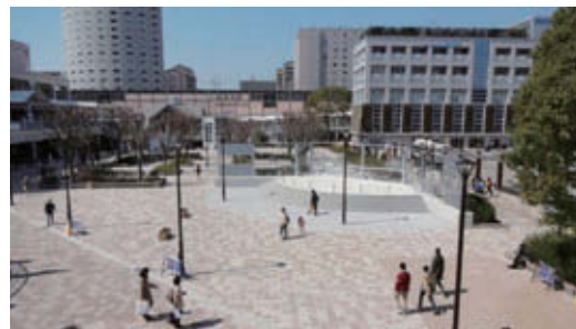
No.9 Road Damage Rehabilitation Works, Restoration and Construction Subsidy
