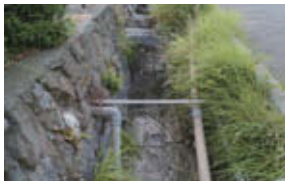
Drainage channels lined with a geopolymer and with cement-concrete
