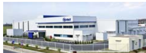
Rodax Vietnam Factory Project
