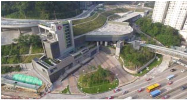
Kwun Tong Line Extension (Contract 1001 – Ho Man Tin Station)
