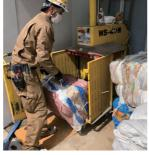
Using a compactor to reduce the volume of waste at the time of disposal
