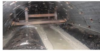
Filling in shield cavities with fluidized soil made from construction sludge
