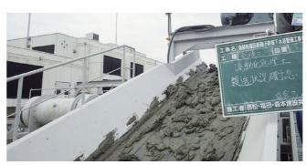
Making fluidized soil using construction sludge generated during shield tunneling
