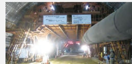
Automated set up of tunnel lining forms
