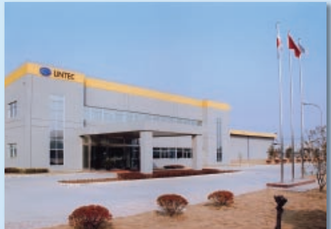
Lintec Suzhou Factory, China
