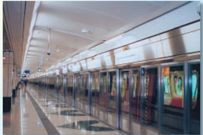
KCRC Contract HCC-300 — Tsim Sha Tsui East Station and Subway, Hong Kong
