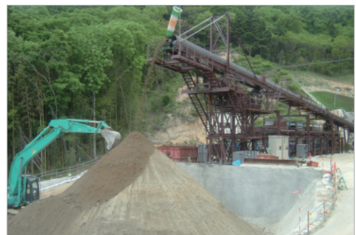
Removing dirt from a tunnel by conveyor belt
