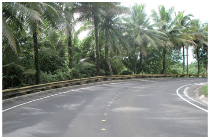
Rehabilitation of Arterial Roads in the Metropolitan Area, Palau
