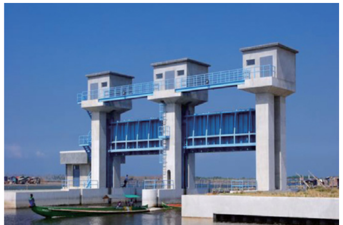
Kamanava Area Flood Control and Drainage System Improvement, Philippines
