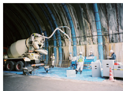
Tunnel lining process
