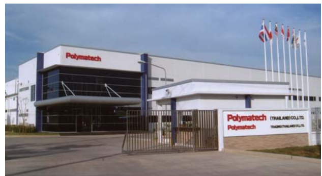
PTT New Factory Project, Thailand
