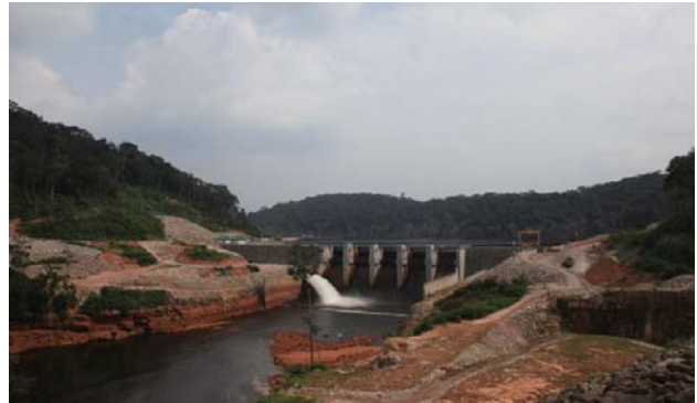
Nam Thuen 2 Hydropower Project, Laos
