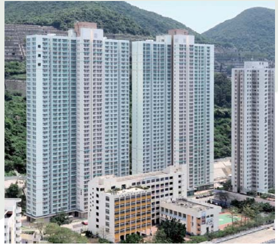
Construction of EX-Chai Wan Estate, Hong Kong
