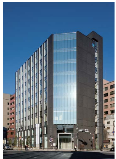
Huric Co., Ltd. Head Office Building
