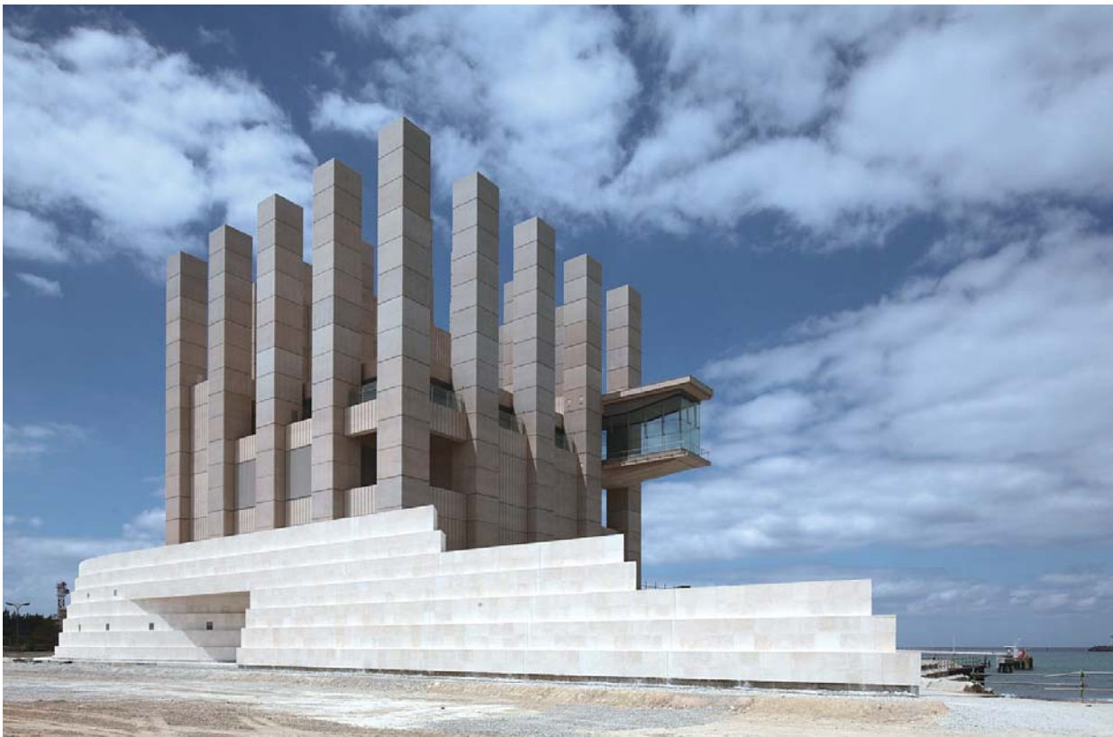
Ventilation Building, Naha Port Freeway Airport Route
