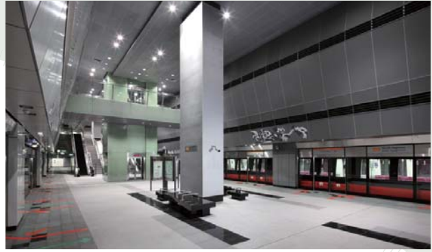
Contract C828, Design, Construction & Completion of Stations at Nicoll Highway & Boulevard including Tunnels, Singapore
