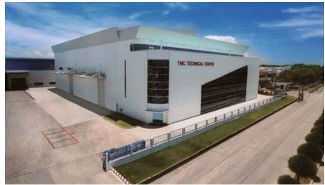
TMC Technical Center Project, Thailand
