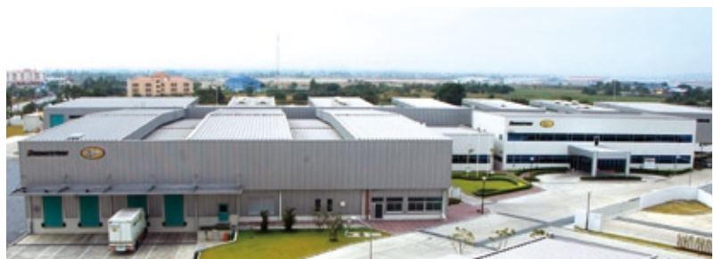
BBMT New Factory, Thailand
