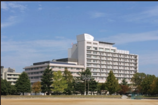
Municipal Hospital (South Wing) Reconstruction
