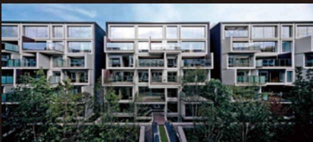
Building Construction, Shibuya Uguisudanicho Plan
