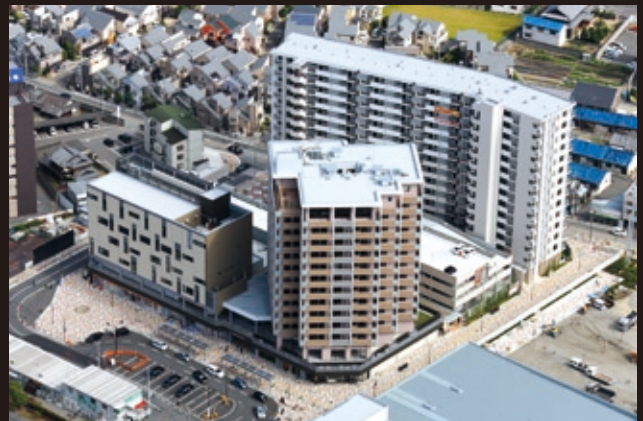
"C" Area Construction, Higashi-kishiwada Land Adjustment Plan for Disaster Prevention
