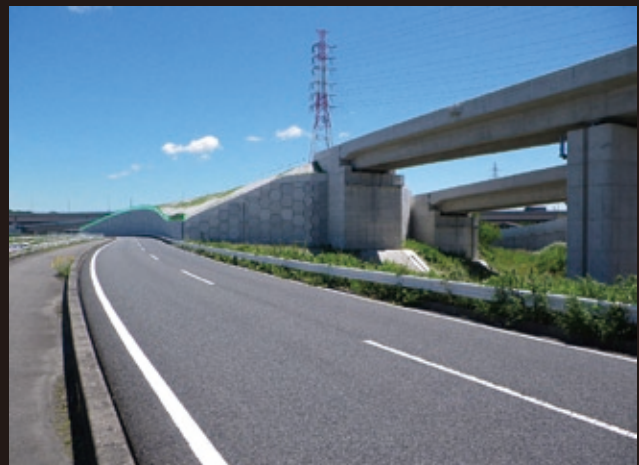
Substructure for Tokai Junction, 2nd Tomei Expressway
