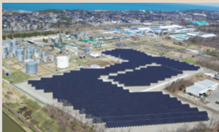
INPEX Mega-Solar Power Station Joetsu Construction
