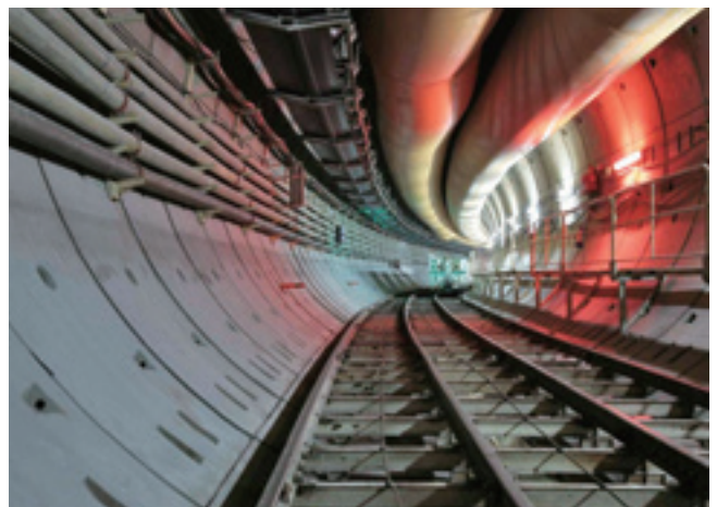
Hong Kong West Drainage Tunnel (Hong Kong)
