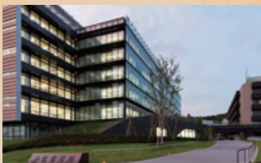
Architectural Work, New Governmental Building Construction, Komaki Municipal Government
