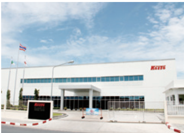
Thai Koito Technical Center (Thailand)
