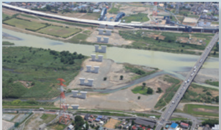
Sagamigawa River Bridge and Other 5 Bridges Construction (Substructure Construction), Shin-Tomei Expressway
