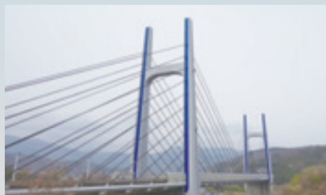
Tomei Ashigara Bridge Rehabilitation Work, Tomei Expressway
