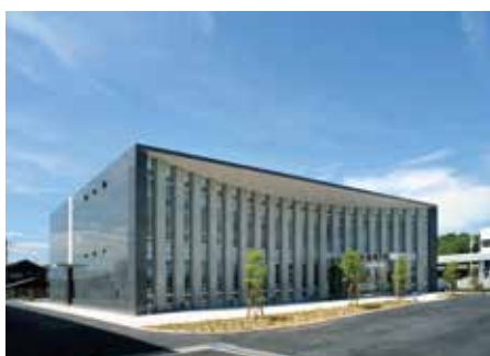
Senbakasei Head Office Building Construction
