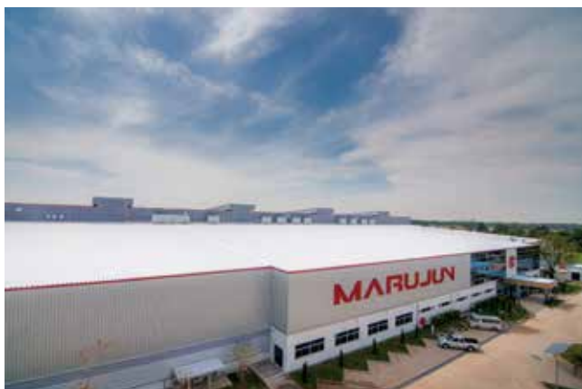
Thai Marujun New Factory
