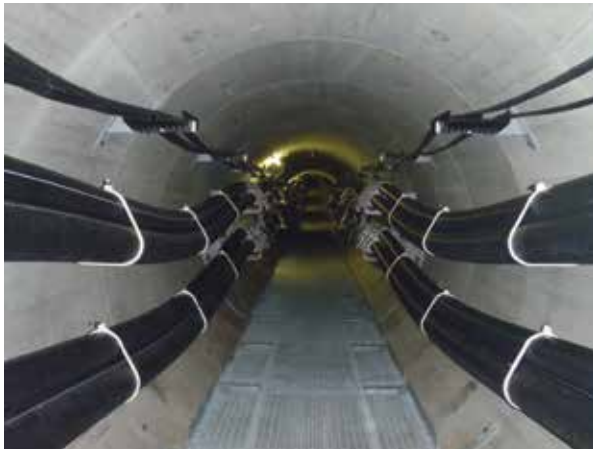
Abekawa River Crossing Tunnel Construction, Surugahigashi Shimizu New Cable Route Construction
