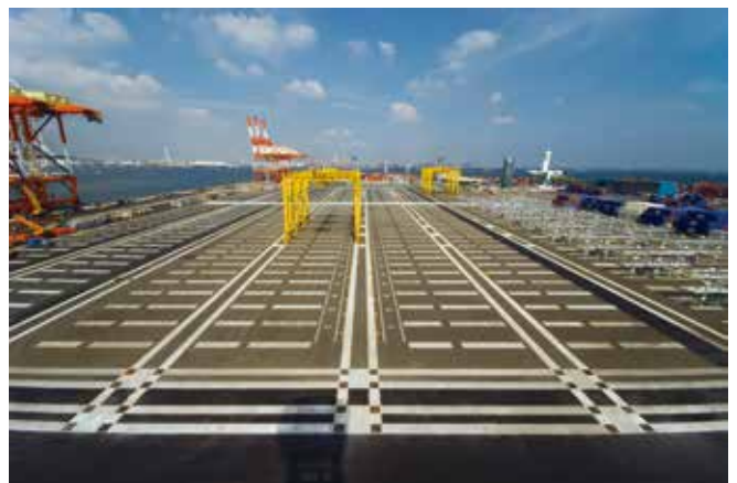
Redevelopment Work for Container Yard, Building and Other Facilities
