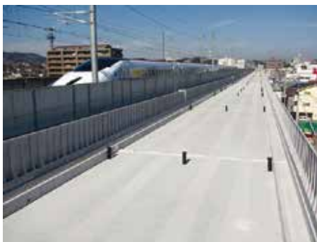
Viaduct Construction, Hanazono Construction Section, Kyushu Shinkansen
