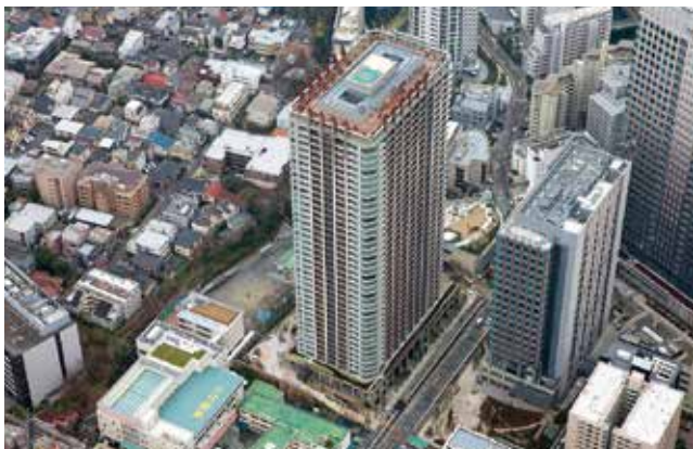
District 1 in Kitashinagawa 5-chome, Urban Redevelopment Project Completed: 2015 Location: Shinagawa-ku, Tokyo Purpose of use: Residential Housing, Commercial Buildings, Daycare Facilities, Regional Community Facilities
