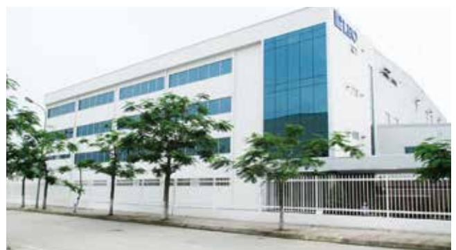
Work of LEO Electronics Vietnam Factory Expansion
