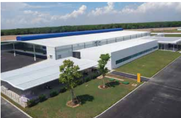
Paramount Bed Vietnam Factory Project Completed: July 2014 Location: Đông Nai, Vietnam
