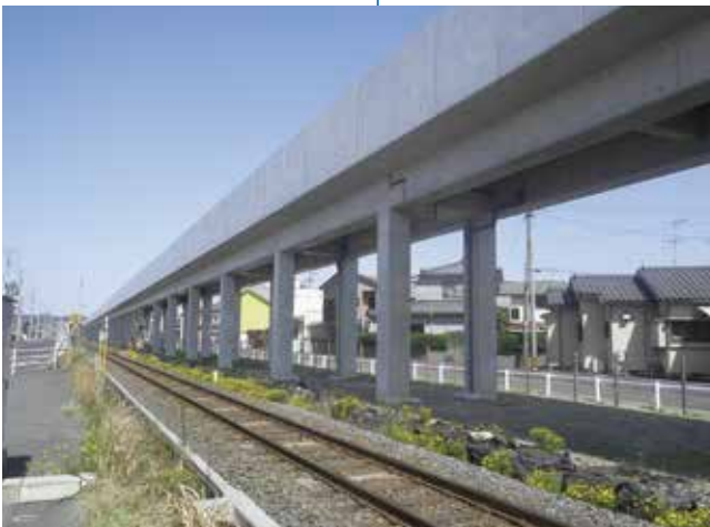
Jinnohira BI New Construction, Taniyama Viaduct, and others Completed: March 2015 Location: Kagoshima-city, Kagoshima Prefecture
