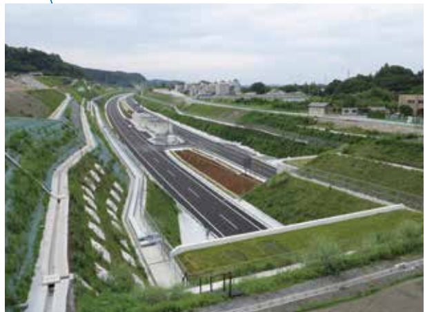
Improvement Work (No. 3 Section), Sumita Mitsukurisan Area, Sagami Longitudinal Expressway Completed: October 2014 Location: Aikawa-machi, Aiko-gun, Kanagawa Prefecture
