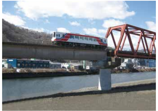
Yoshihama-Kamaishi Section Disaster Relief Project, Sanriku Railway South Rias Line Completed: July 2014 Location: Ofunato-city and Kamaishi-city, Iwate Prefecture
