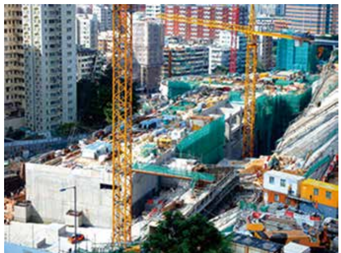
Construction of the Kwun Tong Line Extension Contract 1001
