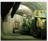
Portable blast protection balloon in use
