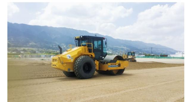
Construction underway using ICT (GNSS\* management of roller compacting)
