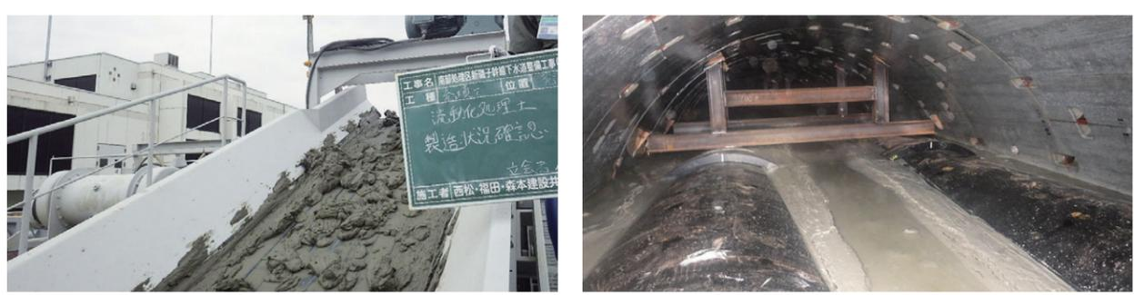
Making fluidized soil using construction sludge generated during shield tunneling
