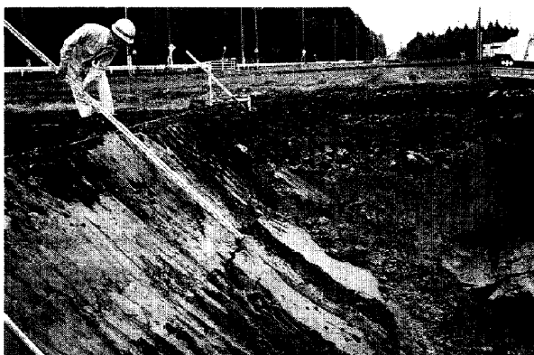
Photo 2 未改良地盤掘削法面(1割勾配)法面亀裂
