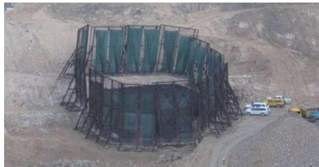
写真-2 発破防護 (Cage+Screen方式)
