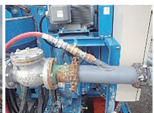
写真-5 鞘管設置
