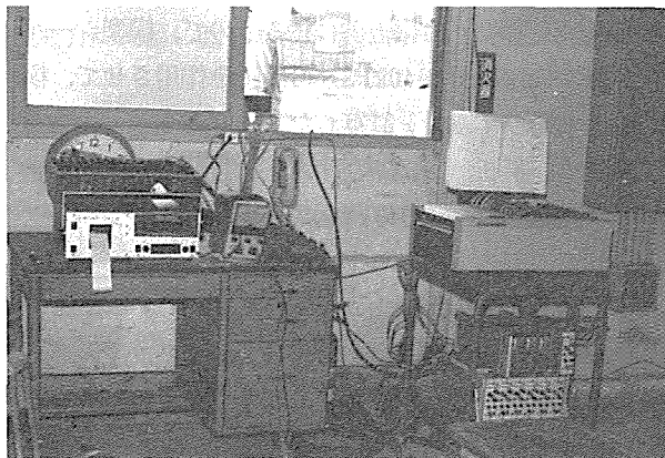
Photo-3 計測装置 Measuring apparatus
