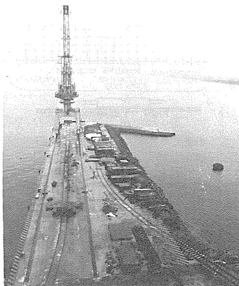
Photo-1 完成全景 Overall view (completed)
