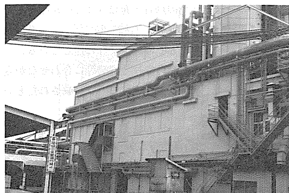
Photo-6 補強改修後の建物全景 Appearance of the structure after reinforcing and repairing
