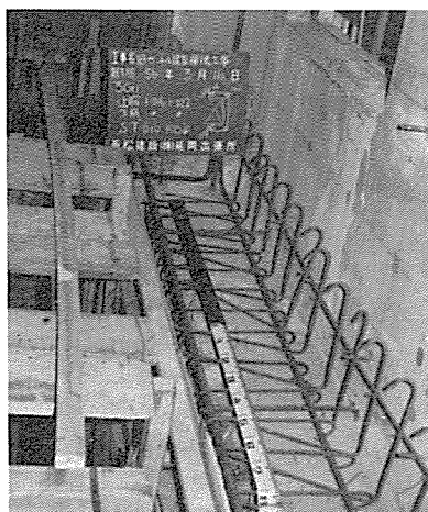
Photo-3 梁の補強筋 Reinforcing bars of girder
