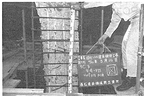
Photo-4 柱の補強筋 Reinforcing bars of column
