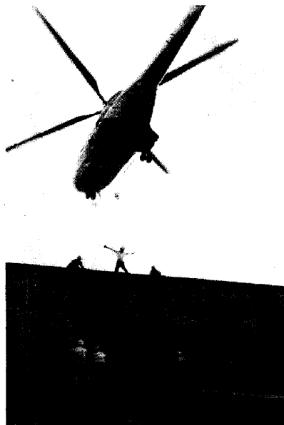
Photo 3 架台鉄骨取付
